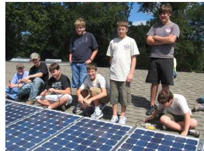
Students installing the modules
