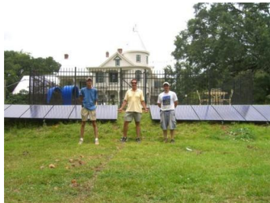
Installation team in front of 2kW system Photo by Jeff Shaw
